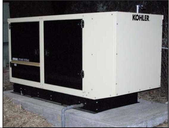
The recent installation of this heavy-duty emergency generator outside MacQueen Hall will now allow borough residents to use the building as an emergency shelter in the event of a widespread disaster. The powerful 60KW/75K, 120/208 volt, three-phase generator has already been tested, restoring power within 6 seconds of a test outage.
