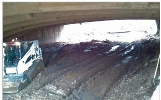
**Work under the bridge also included the removal of 500 cubic yards of silt, using a small bulldozer.**
