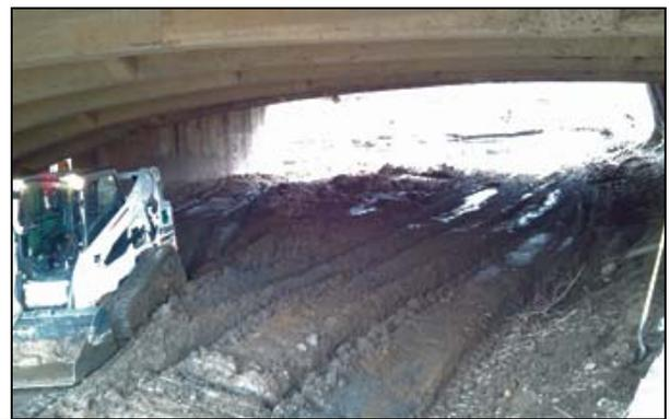
**Work under the bridge also included the removal of 500 cubic yards of silt, using a small bulldozer.**
